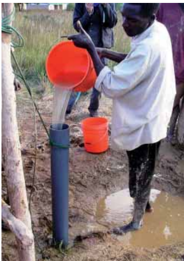
Flushing the well with water
