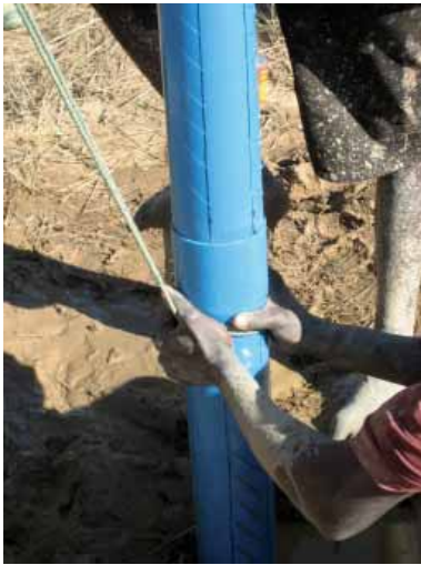
Use of rope during installation
