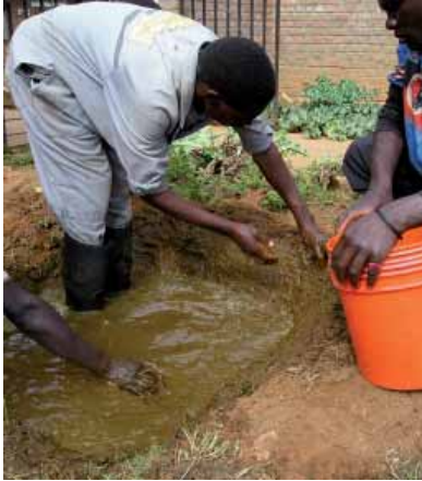
Mixing cow dung with working water
