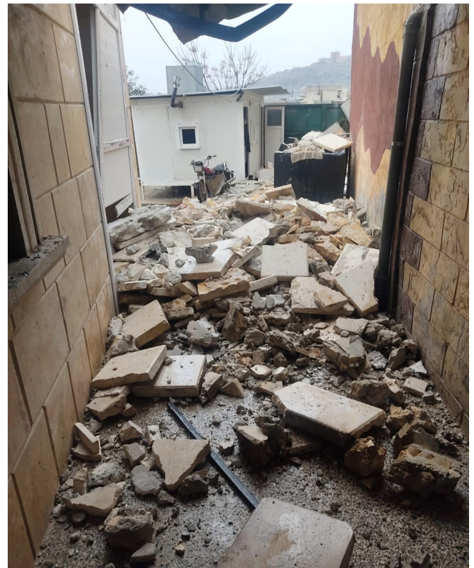
Destruction at RI's one-stop center in Sarmada, Northwest Syria.
