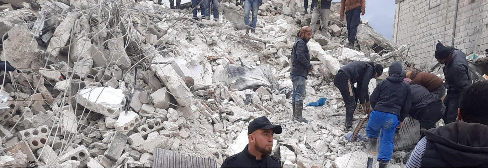
Rescuers working to rescue persons from underneath the rubble in Harim, Northwest Syria.
