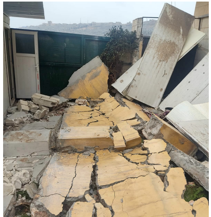
Destruction at RI's one-stop center in Sarmada, Northwest Syria.
